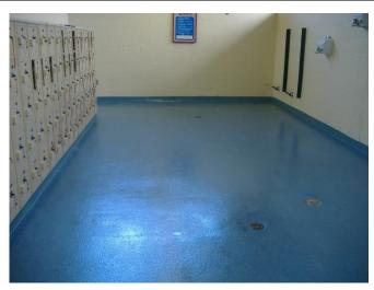
Preparation Guide. A minimum surface profile of CSP-2 is acceptable in some cases, but a shot-blast CSP-3 profile is strongly recommended for most applications.
