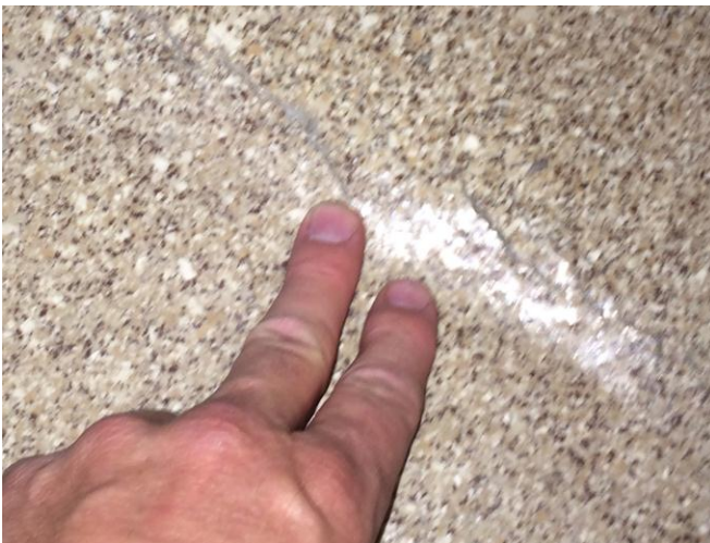
Figure 4. This crack is over a contraction joint where the substrate continued to shrink. When the substrate expands a hump will be evident as the material is forced upward.
