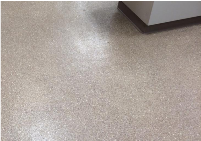
Figure 4. This crack is over a contraction joint where the substrate continued to shrink. When the substrate expands a hump will be evident as the material is forced upward.
